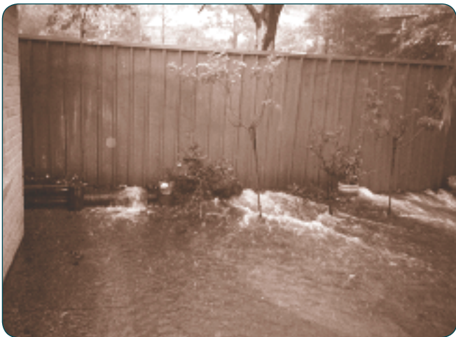
Serious flooding as the result of inadequate drainage – see case study 20 for details
